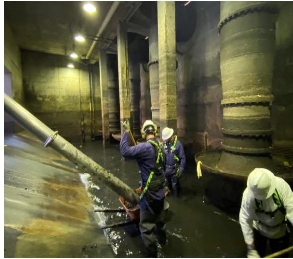
J-2 Pump Station Desilting
