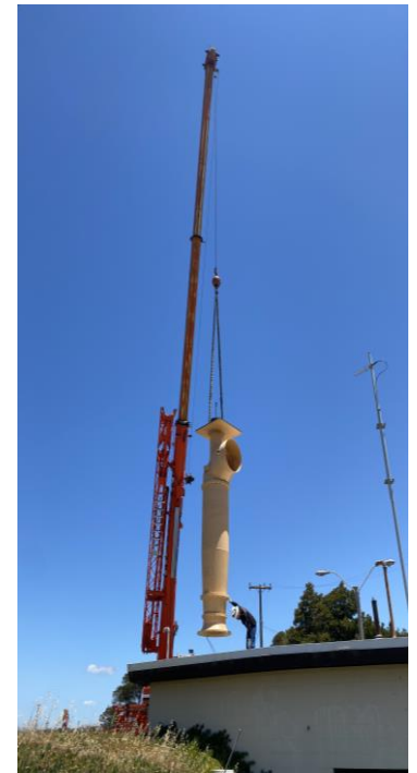
Pump Overhaul and Install at Alvarado Pump Station
