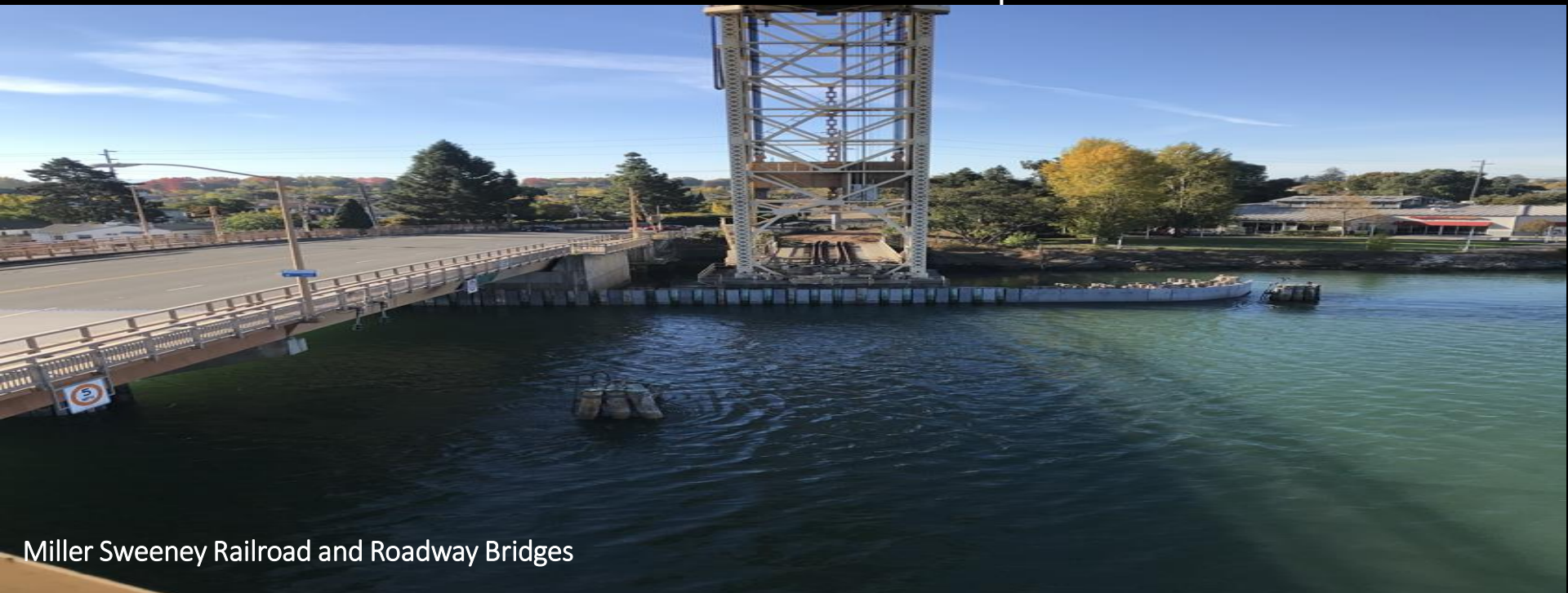
Park Street Bridge
